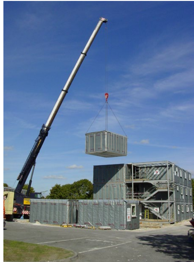
ABOVE Stacked modules mid-construction
